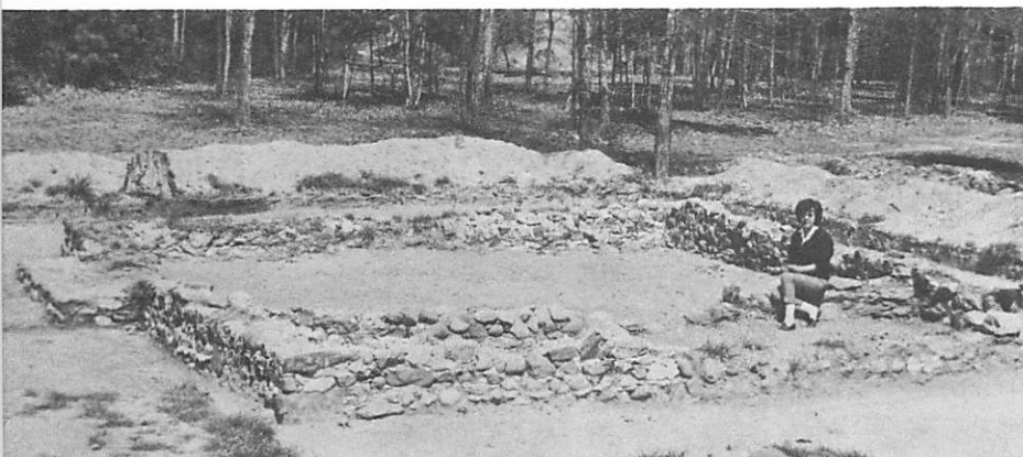
Excavated Courthouse Ruin
